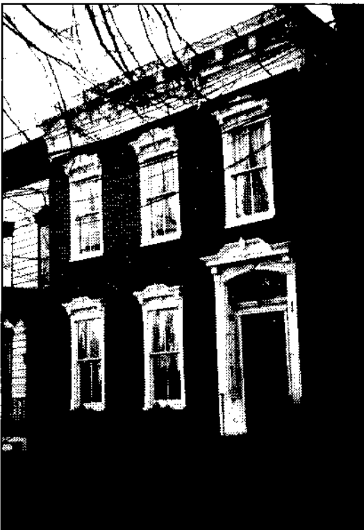
238 Green Street. Celebrated on the 2005 Walkabout, here dressed for the winter with ornamental tree, wreath and window decorations.
