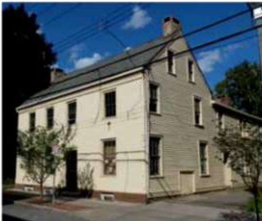
The Jemie Boyd/Issac DeGraff House 14 North Ferry Street Work-In-Progress, Owner, Robin White
